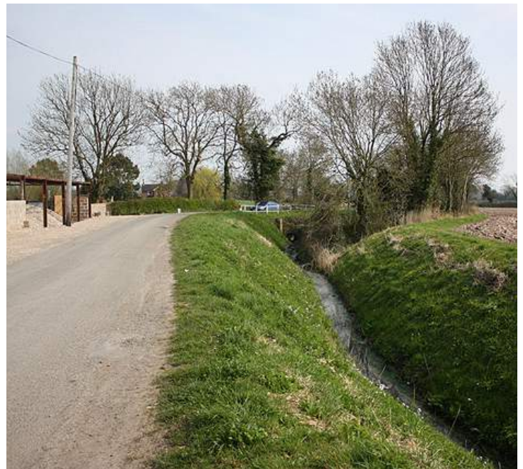
Example diversion ditch ( https://geograph.org.uk/ )
