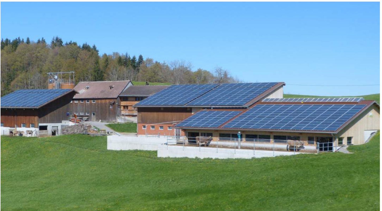
Solar arrays on agricultural facility
