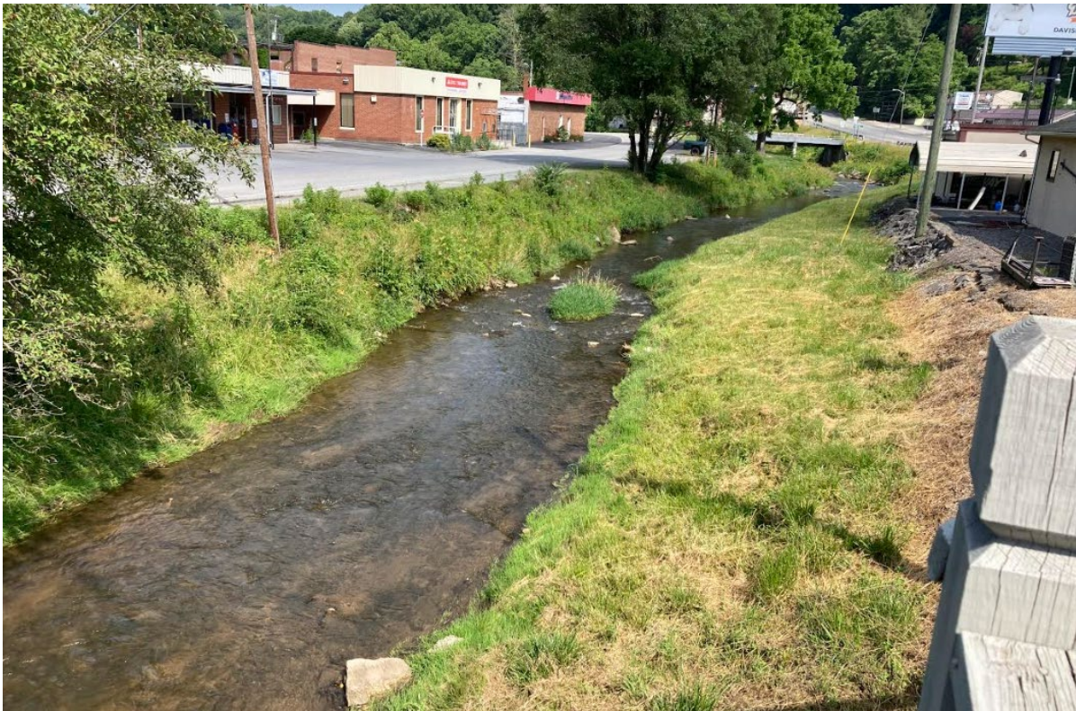
Maggodee Creek from Boon Street looking towards Main Street (on the left) and Church Hill Street (far bridge)
