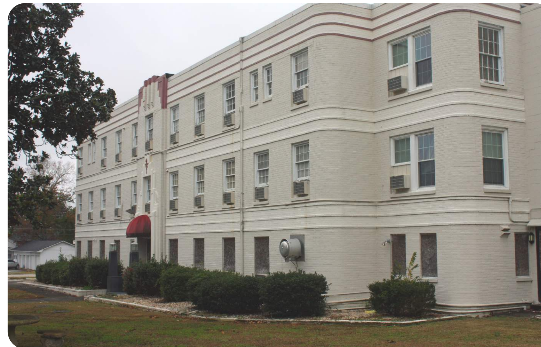
Former Betsy Johnson Memorial Hospital in Dunn is an architecturally and culturally significant landmark that offers many options for rehabilitation and reuse.
