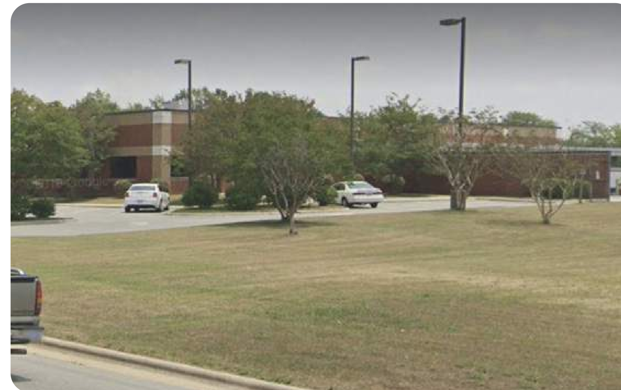
Typical Existing Gateway into the City of Dunn
