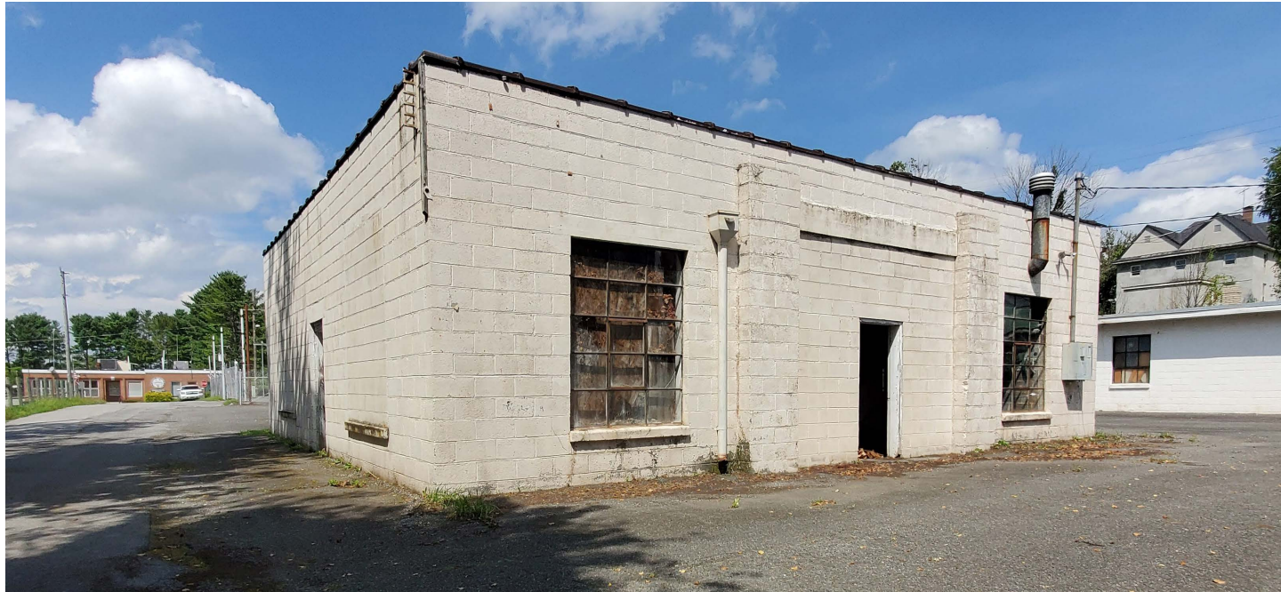
Exterior of Laundromat building on site
