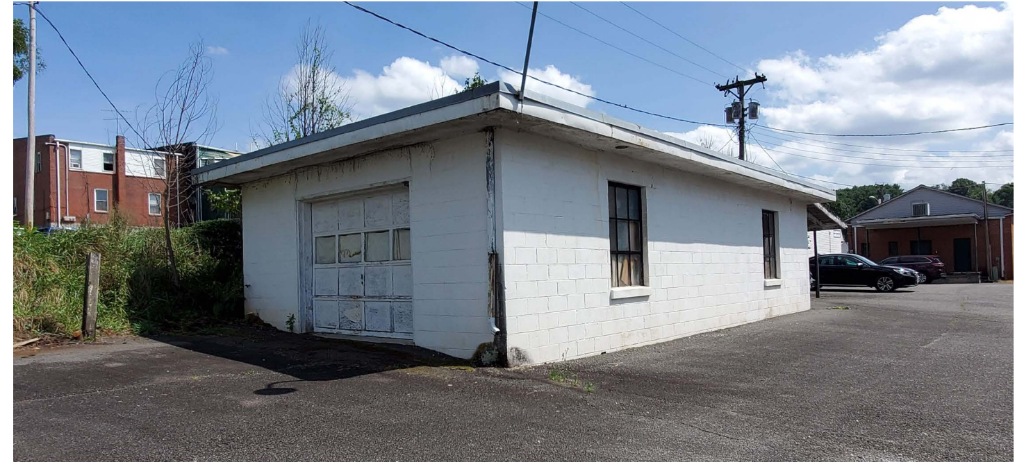
Exterior of auto-shop building on site
