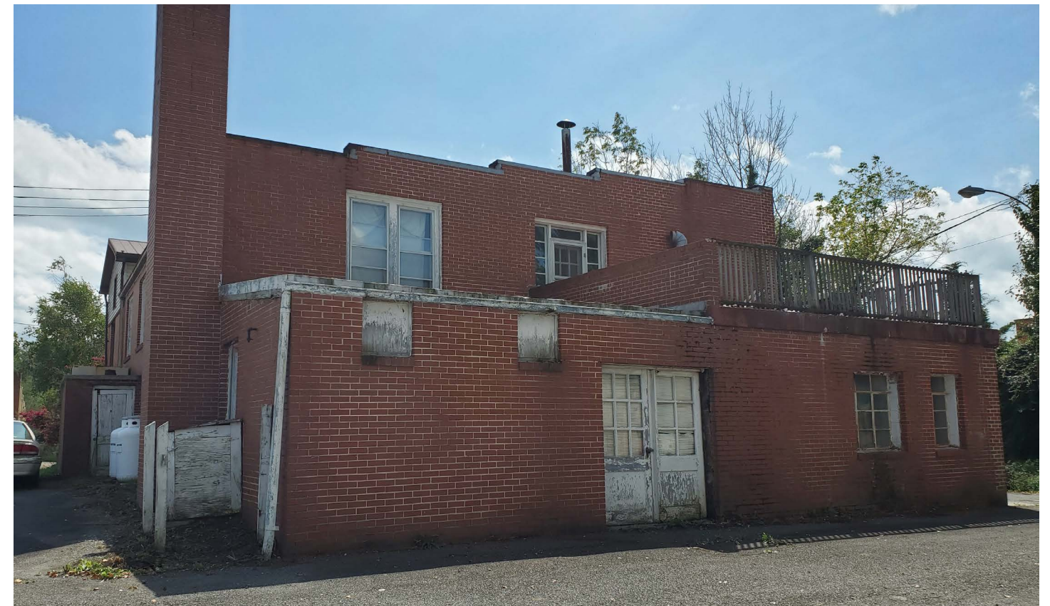
Exterior of the Harris Cleaners Building on site
