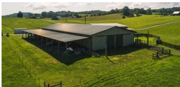
Barn This 300x140 s.f. roofed barn with 50x60 s.f. shop containing a concrete floor, electricity, doors and insulated roof. The barn has a working cattle headgate and area for equipment storage. It is surrounded by feeding troughs and 7 miles of fencing.
