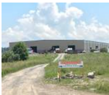
Construction in Progress on Industrial Facility at Southern Gap
