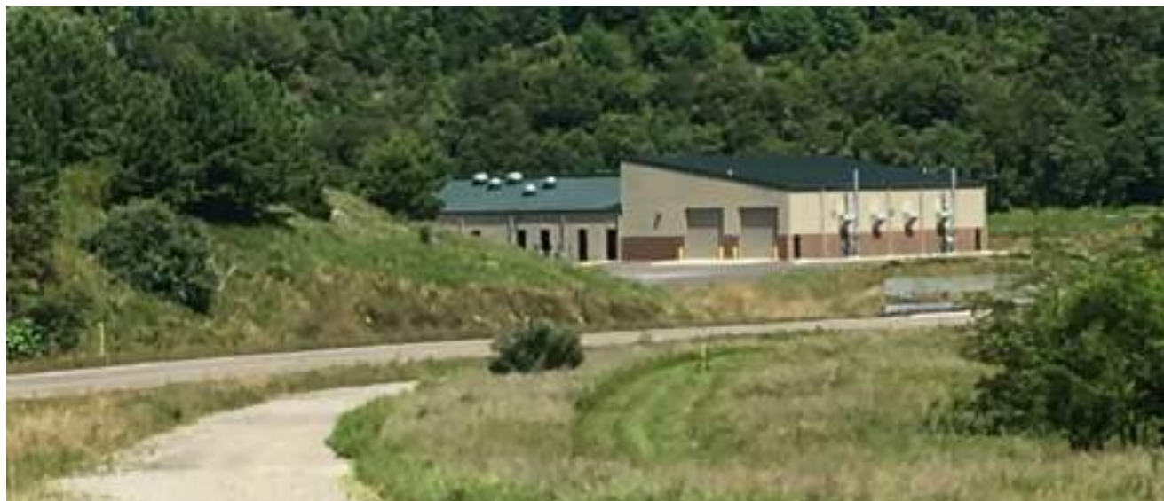
Recently Constructed Transportation and Logistics Center
