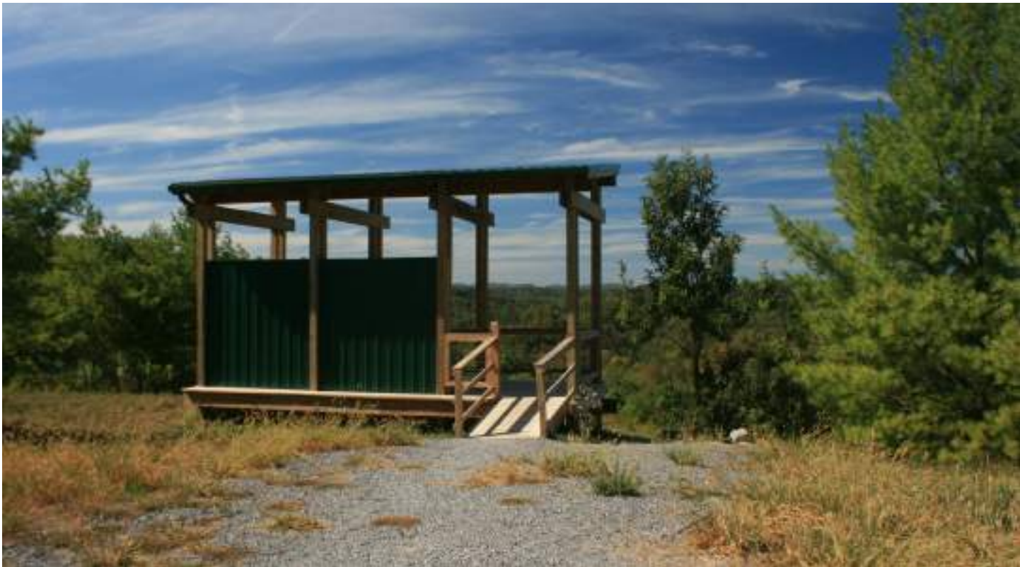
Wildlife Viewing Shelter overlooking the Elk food plots below
