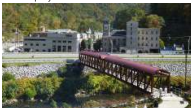
Pedestrian bridge across the Levisa River connecting the new Grundy Town Center to the Courthouse Photo credit: VirginiaPlaces.org
